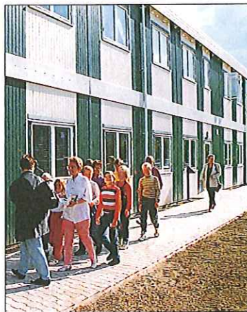
In ten days, SektionsByggarna delivered and assembled an eight-classroom school in Ribnitz, northeast of Rostock, Germany.
