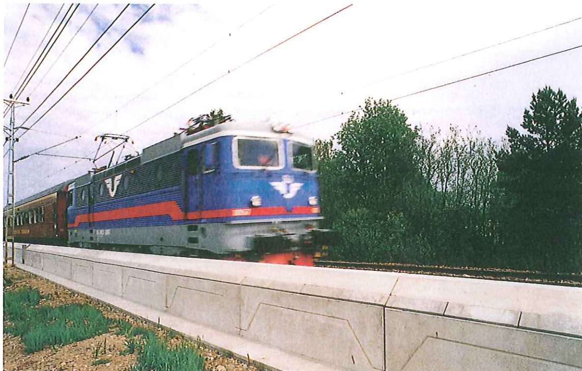
Skanska Prefab's Soundtrack noise barrier does not block the view and cuts the noise from high-speed trains by nearly half.
