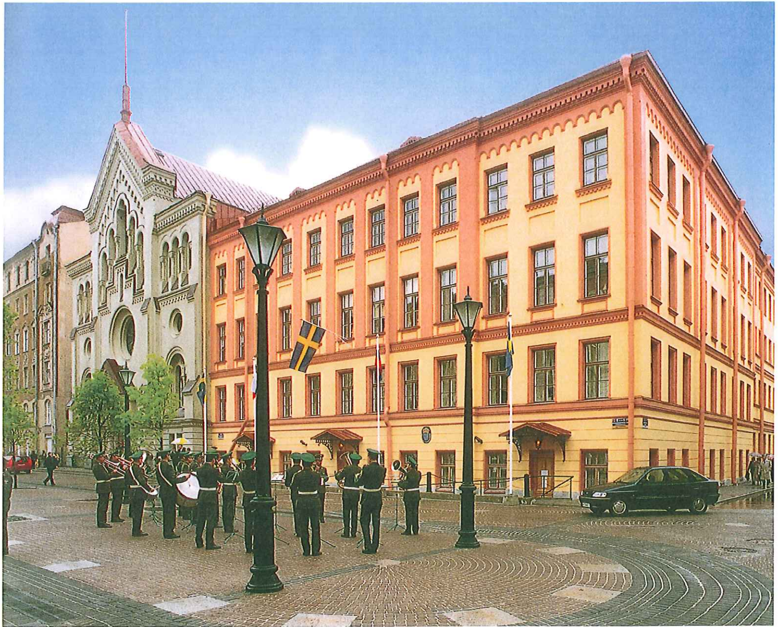
Sweden House, a 19th century building in central St. Petersburg, Russia with historic landmark status, was refurbished inside by Skanska into a modern office building.
